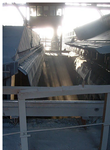
Figure 1. Dust generation during the unloading of a dump truck into the feed hopper of a cone crusher Source: compiled by the authors
